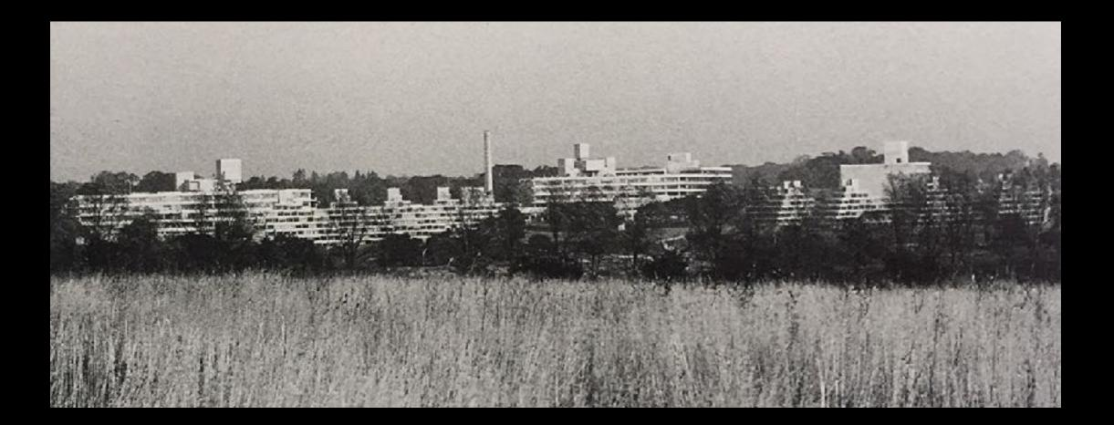
...the speed of student intake demands use of systems for quick construction. buildings are made from large repetitive precast elements manufactured under controlled conditions on the site or in a factory and dry assembled...
